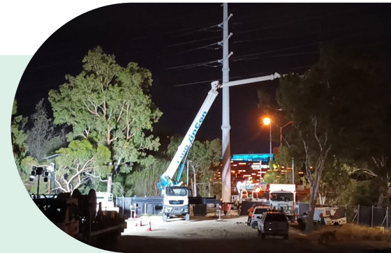
HV pole installation by Western Power
