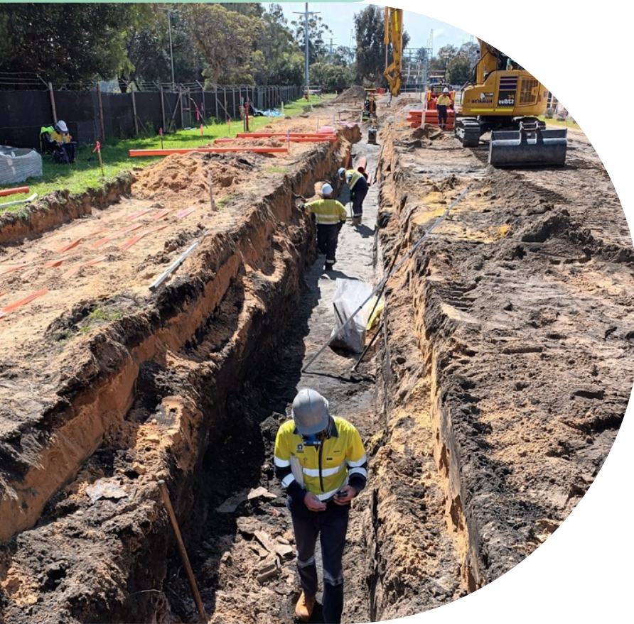
Installation of underground power services along the Swan River foreshore
