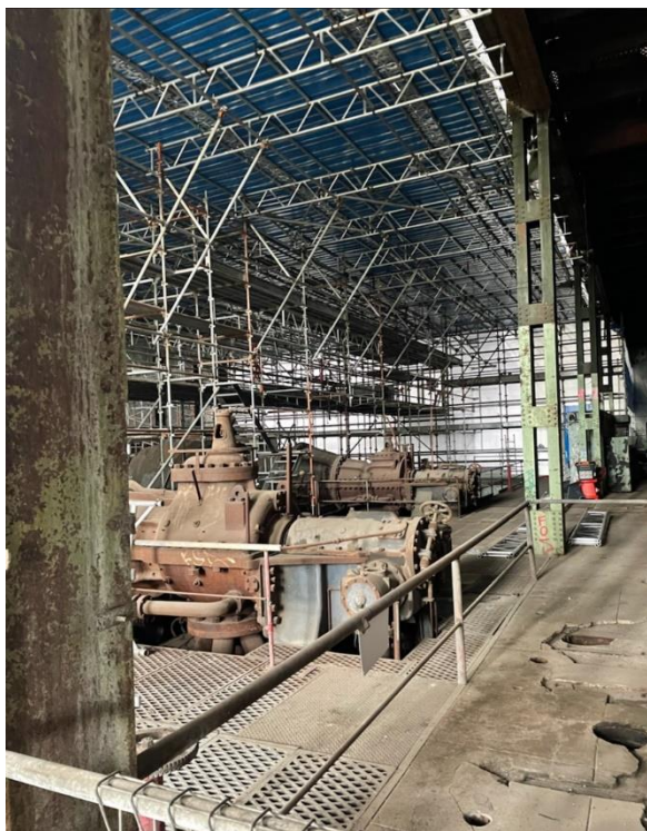
Above – Scaffolding to access the work areas inside the Power Station building
