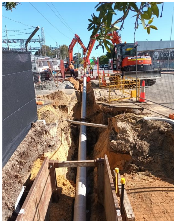
Above – ATCO installing new gas infrastructure under Summers Street
